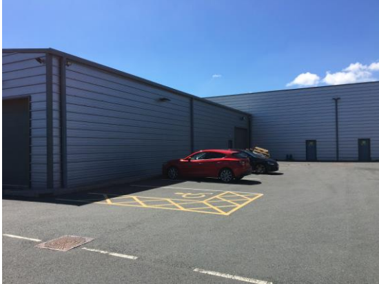
Unit 3 External showing parking area
